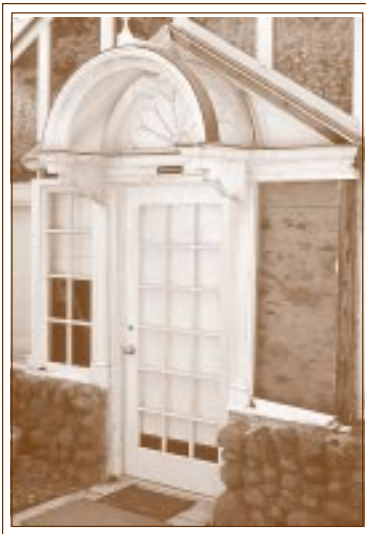
Restoration of greenhouse door in progress.
